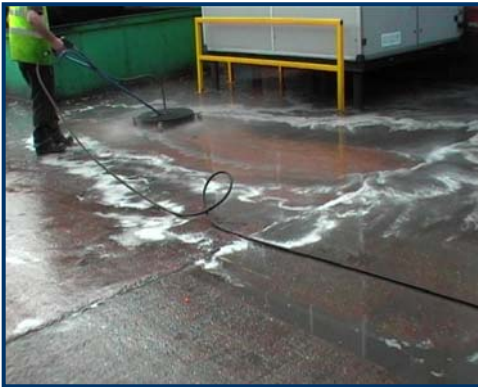
Cleaning by pressure washer
