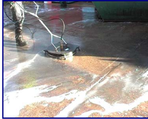
Pressure washer cleaning
