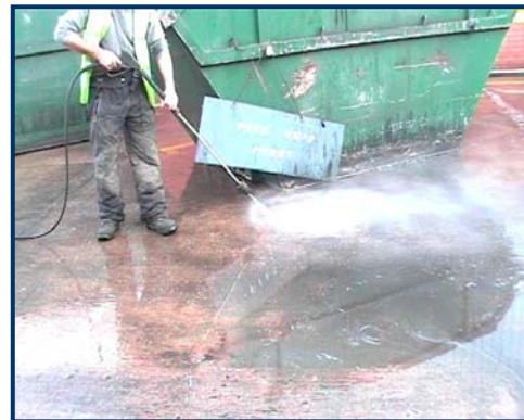
Pressure lance cleaning
