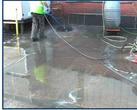
Cleaning by pressure washer
