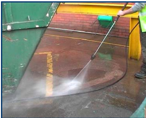
Pressure lance cleaning
